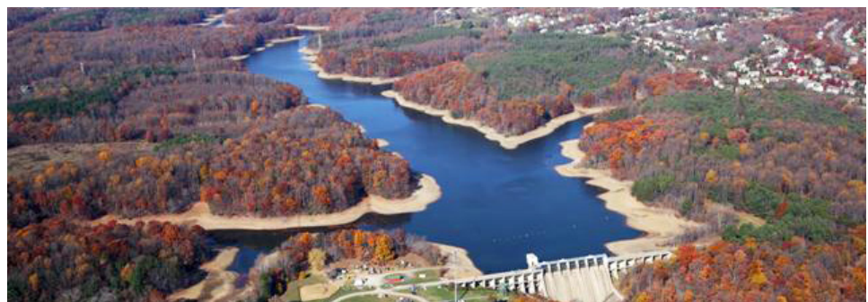
Washington Suburban Sanitary Commission’s T. Howard Duckett Dam on Rocky Gorge Reservoir, Howard and Prince George’s Counties
